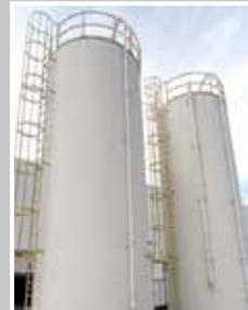
View of Silos
