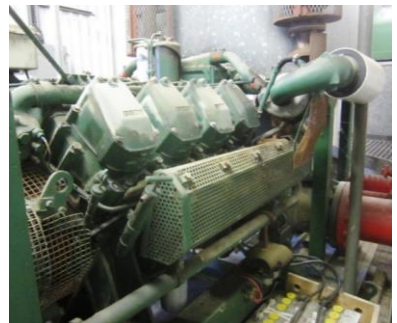
Sigmund Pulsometer fire engine pump with Fiat engine (2-off)
